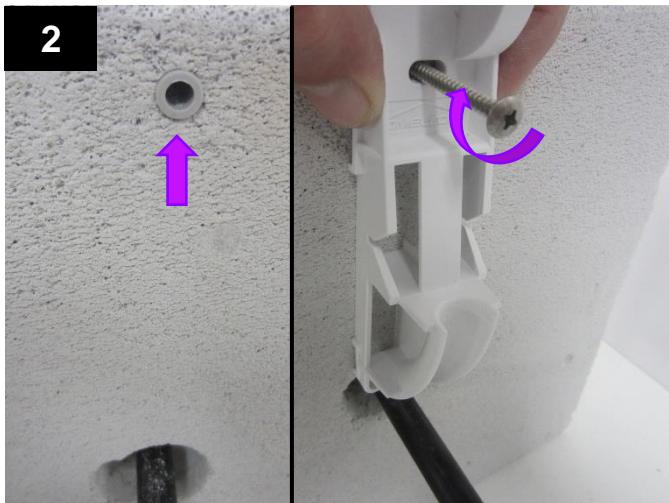
Secure the base with the screw and plug supplied.
