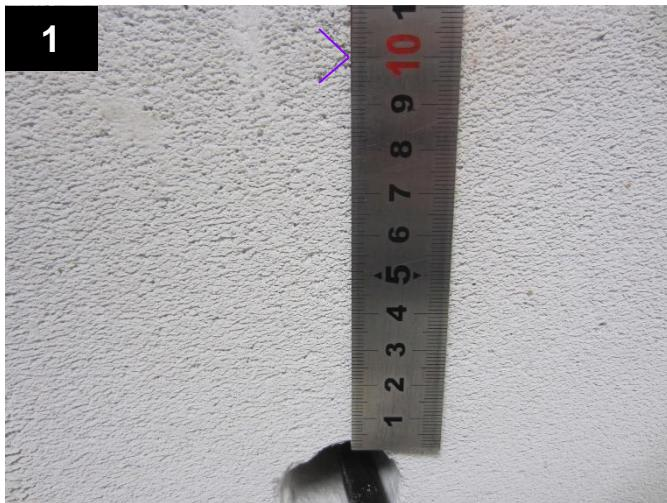
Drill the fixing hole, Ø6mm, 10 cm from the edge of the through hole in the desired direction of curvature of the cable.
