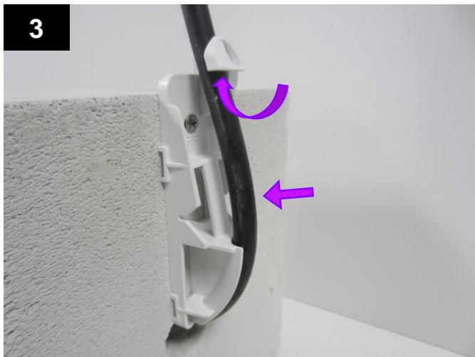
Pass the cable under the hook.
