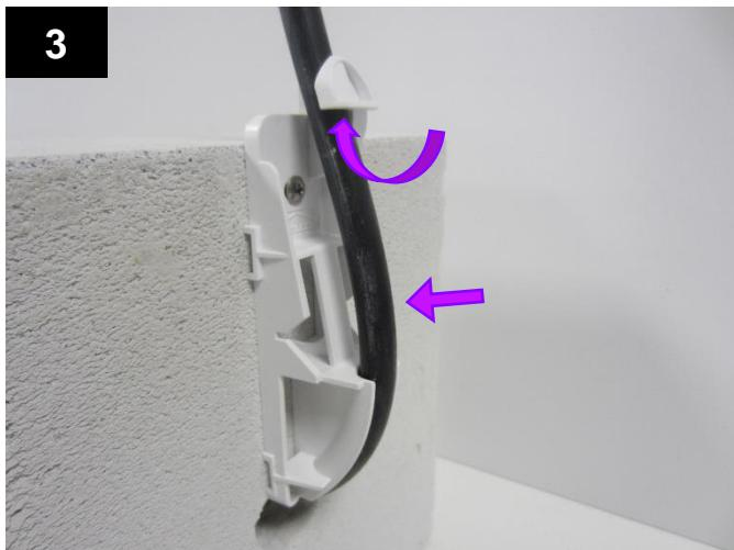
Pass the cable under the hook.
